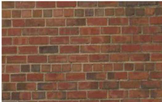
Five course American Brick Bond masonry walls
