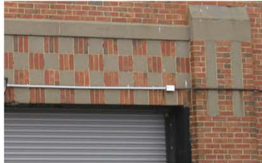
Garage doors w/ concrete capped pylons + Checkerboard Brickwork
