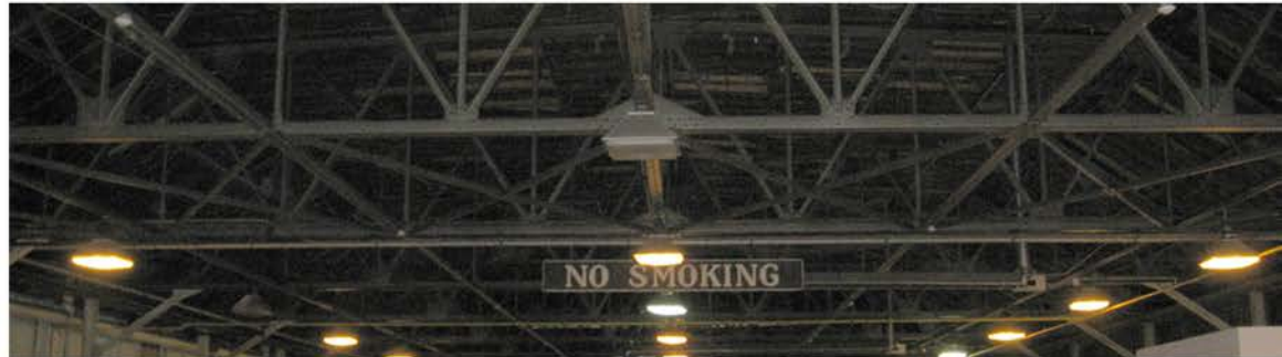
steel truss structural system
