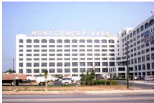
Figure 6: The Montgomery Ward building prior to rehabilitation.
