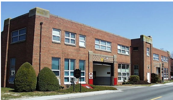
Figure 11: The Motor Pool Building façade from the southwest.
