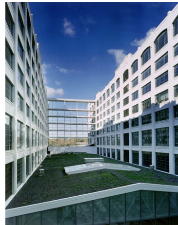
Figure 8: The glass connector between building wings with the green roof in the foreground.
